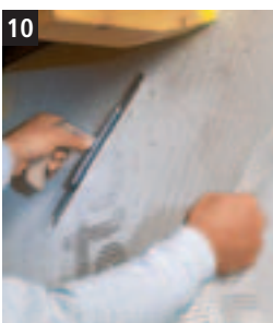
10 Reinforcement Reinforce the entire surface and work the Sto Glass Fibre Mesh into the reinforcing plaster.
