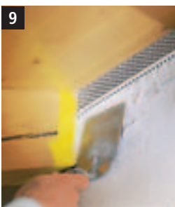
9 Roof Vent Profile Embed the Sto Roof Vent Profile in the reinforcing plaster.
