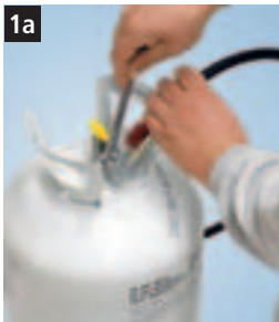
1a Screw Sto-Turbofix cylinder and accessories into place
