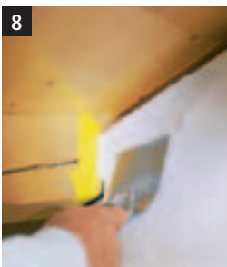
8 Apply reinforcing plaster between the roof rafters.
